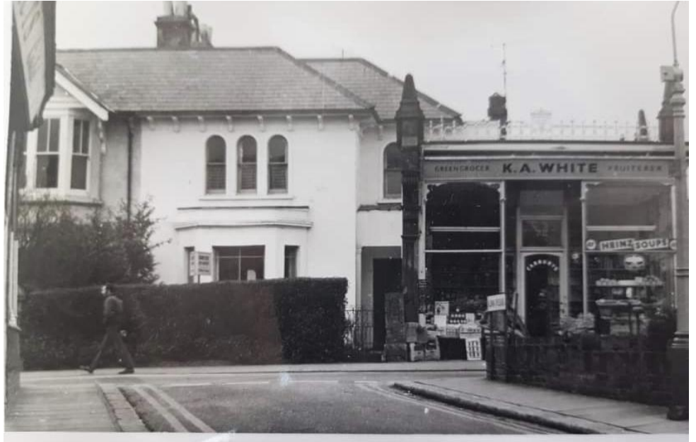
70-72 Sedlescombe Road North 1973. Looking from junction of Alma Villas.
