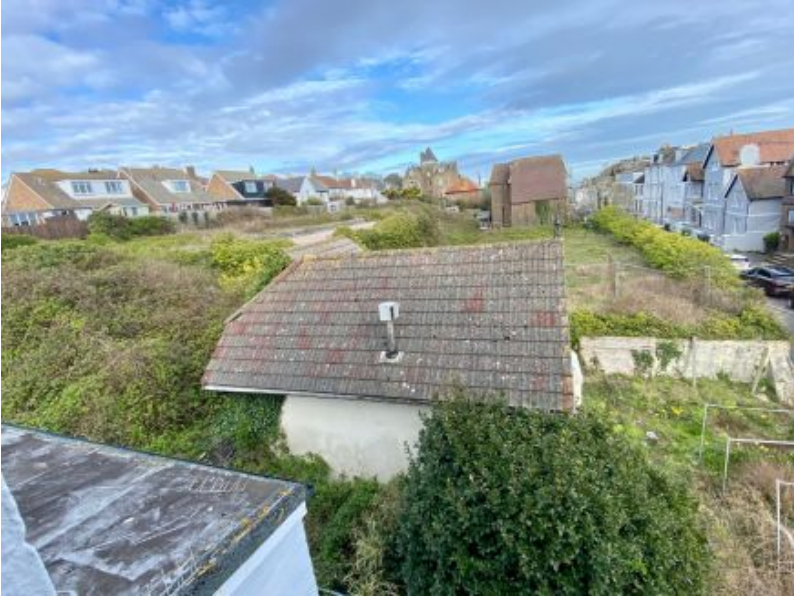
View of the Cottage and Reservoir site
